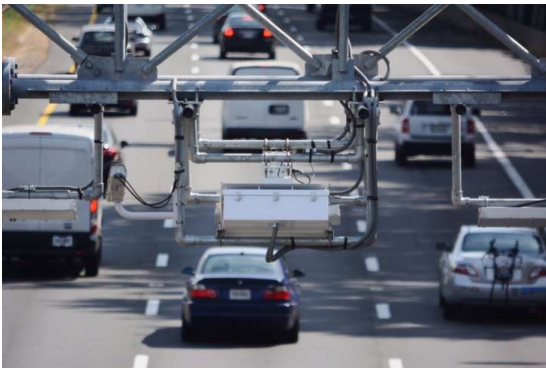
Gantries with electronic tolling equipment
